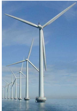
Fig. 1. Rødsand Offshore Wind Farm with 72 Bonus 2.3 MW Wind Turbines on Concrete Gravity Foundations
