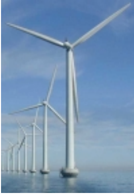
Fig. 1. Middelgrunden Offshore Wind Farm with 20 Bonus 2 MW Wind Turbines on Concrete Gravity Foundations
