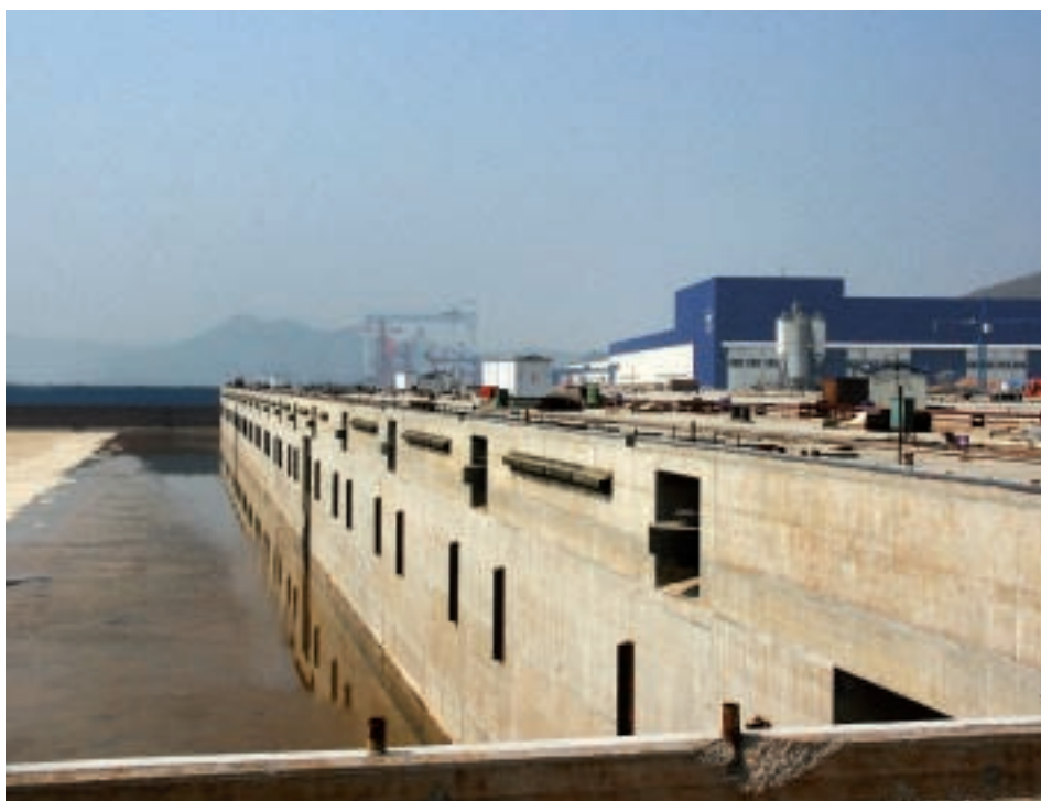
The brand new dry dock at Bohai is 488 metres long, 107.5 metres wide and ready for the construction of some of the world's largest vessels. The water in the dock is from the first flooding to test the dock. Photo: Bohai
